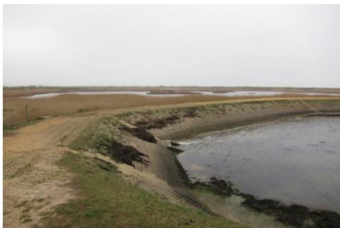
Pennington, view of outflow by survey point.
